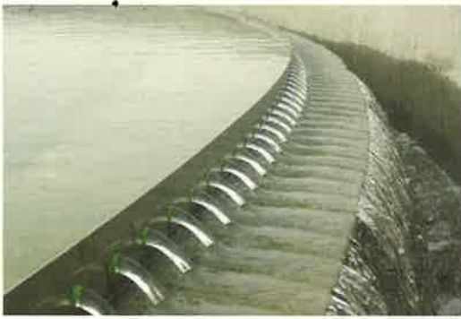
Water Supply & Waste Water
